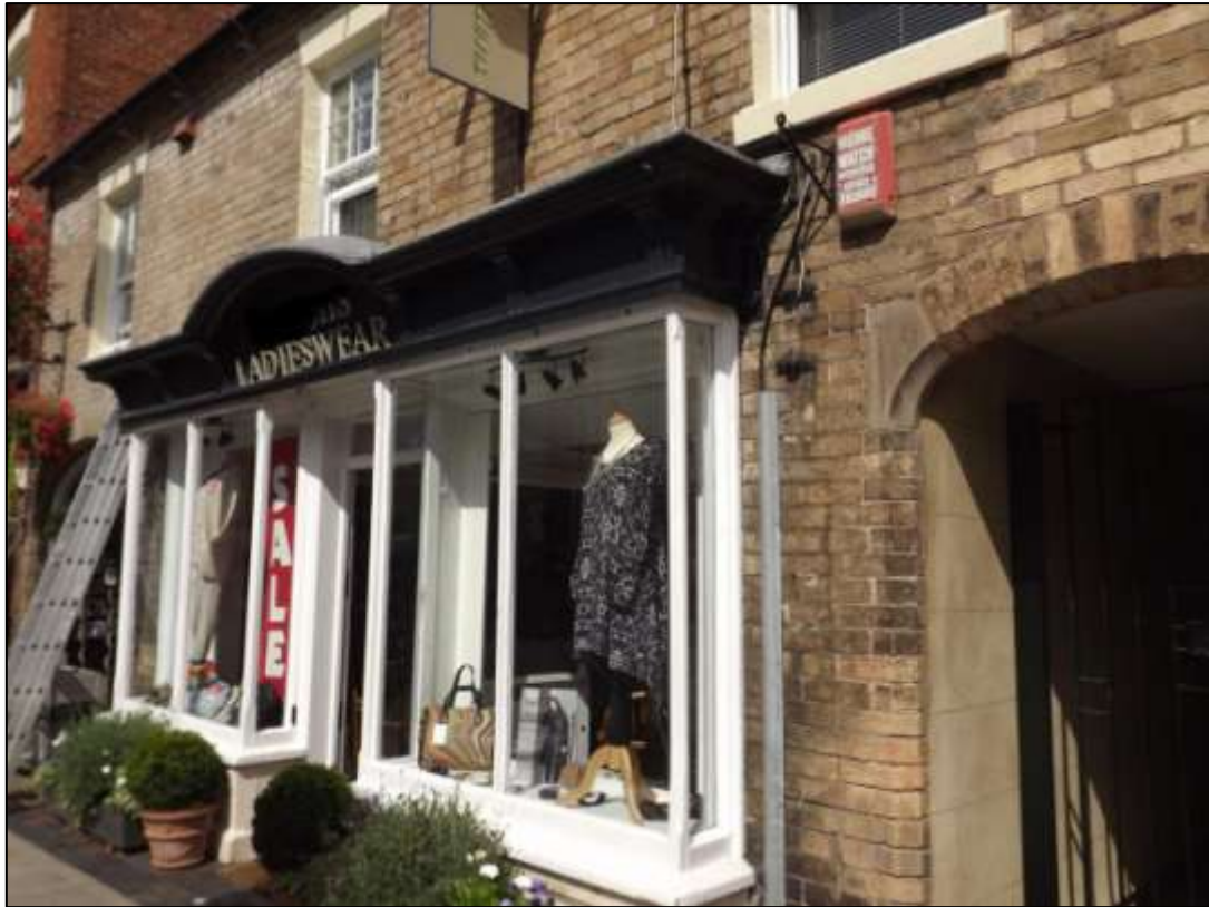
Figure 31 Shopfront at 36 High Street
