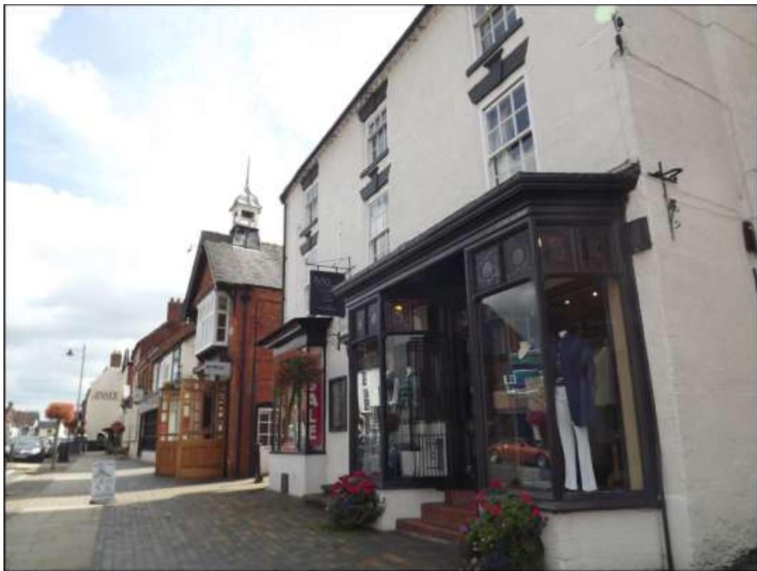
Figure 32 Victorian shopfront at 43 High Street
