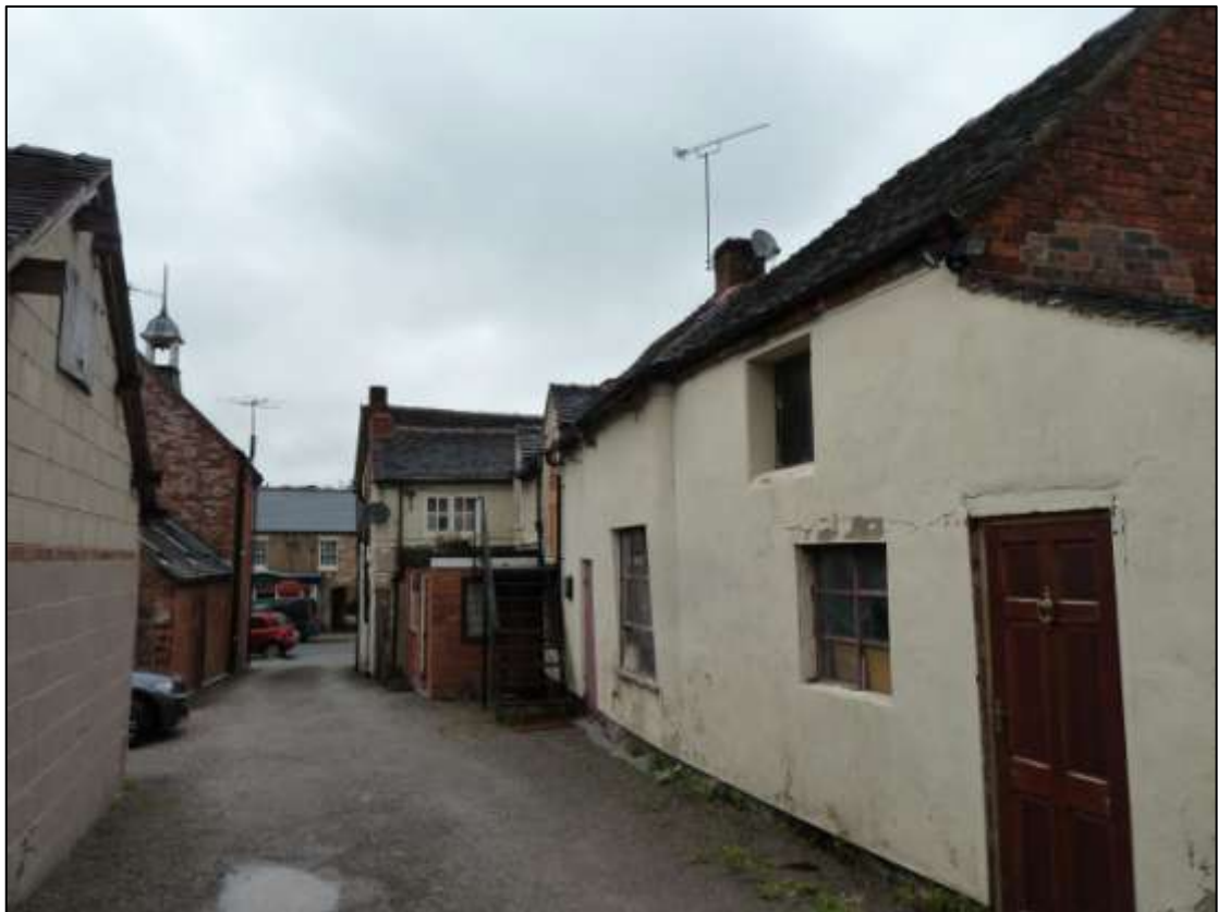
Figure 14 The rear of 35 High Street, which may have medieval origins. Although the building has suffered modern accretions, the burgage plot and character of the building remain.
