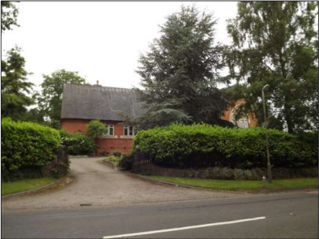
Figure 48 The former Memorial Hall by G.E. Street
