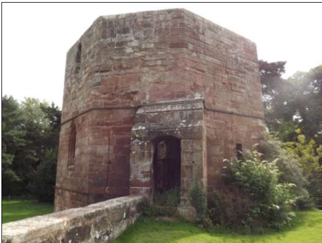
Figure 51 14th century tower at Eccleshall Castle
