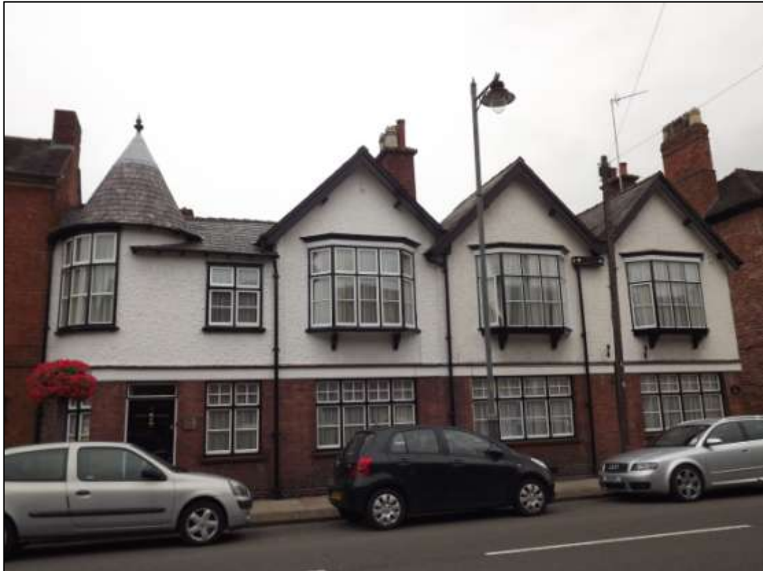
Figure 12 50-52 High Street, the gables and turret facing High Street were added in the early 20th century
