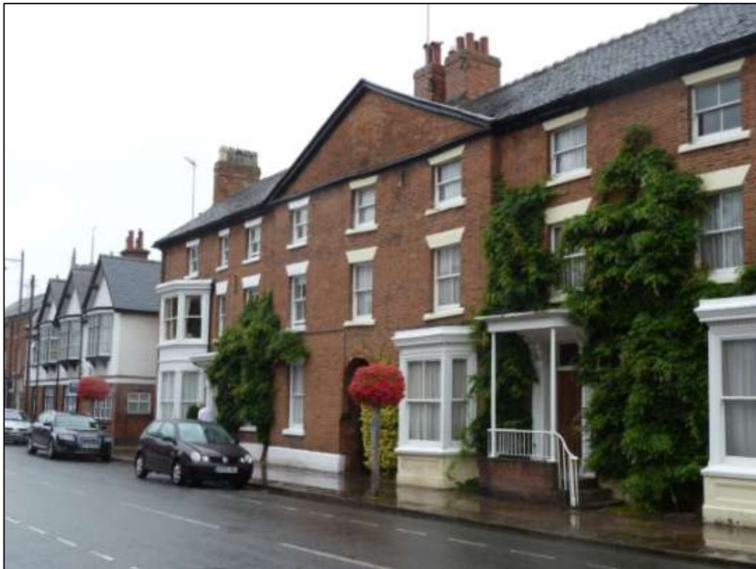
Figure 10 46-48 High Street has a strong visual presence in the street scene. Properties on High Street generally front onto the pavement.
