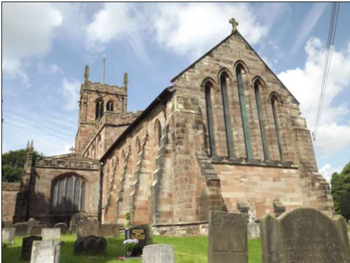
Figure 52 The lancet windows in the east wall are by G. E. Street
