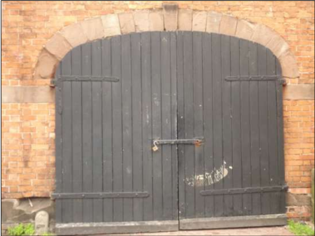
Figure 24 The cart entrance at The Kings Arms with sandstone depressed arch and original L-shape strap hinges
