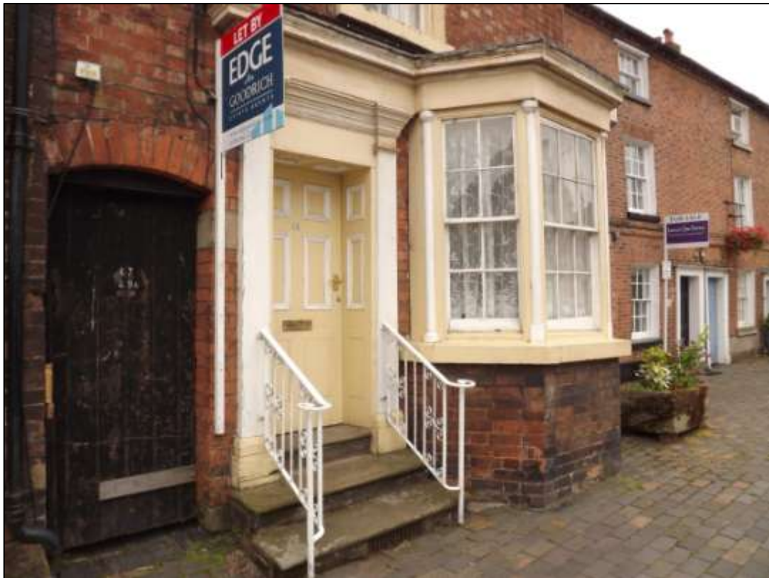
Figure 22 Plank door leading to former burgage plot, early 19th century door with Bolection moulding and canopy, and canted bay window at 47-49 High Street, and door surrounds with flat canopies at 51-55 High Street (far right)
